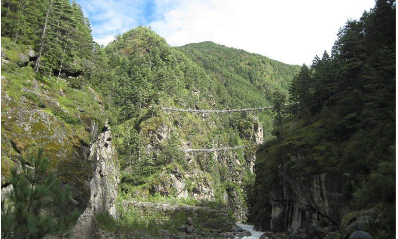
Spectacular Larcha Dovan Footbridges
